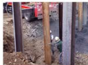
Insert H beam into the drilled hole
