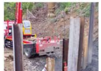
Insert H beam into the drilled hole
