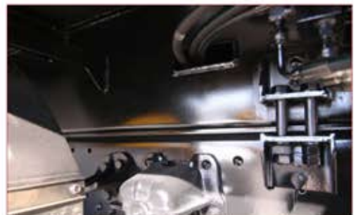
Upgraded Sub-frame Reinforcement
