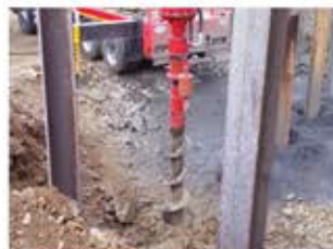
Withdraw screw by air blowing
